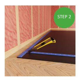
Cut NuWave<sup>™</sup> Base to size using a straight blade cutting tool with a t-square to ensure it is straight.
