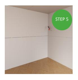
Install your plasterboard over the NuWave<sup>(TM)</sup> Base and caulk the seams with an acoustic sealant to achieve the best results before finishing and painting your walls.
