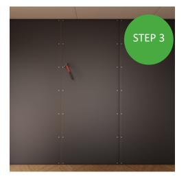
Place the first length of NuWave<sup>™</sup> Base butted up against the ceiling and allow to drape evenly to the floor. Screw, nail or staple into place.
